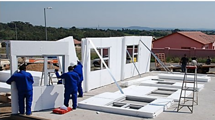
4. Insulated concrete composite (ICC)
