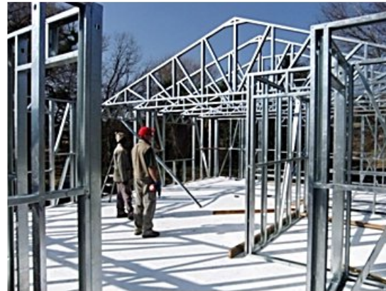
1. Light steel framing
