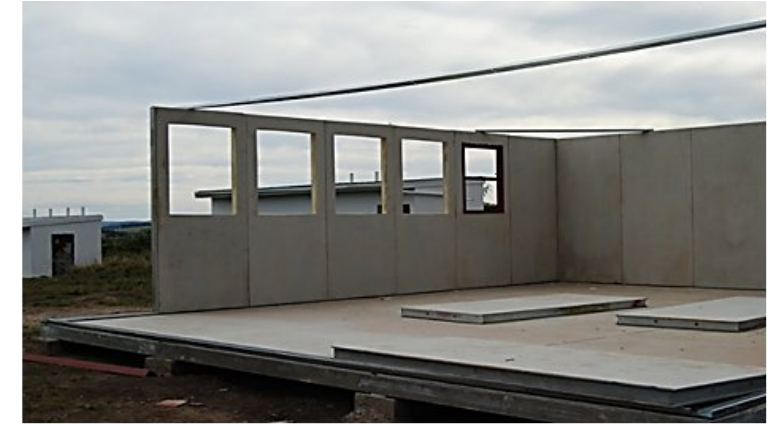
5. Structurally insulated panel
