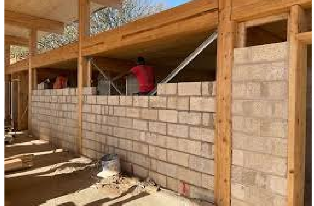
Non-standardised/Innovative (Hempcrete blocks)
