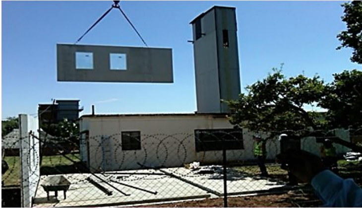
3. Precast concrete sandwich panel
